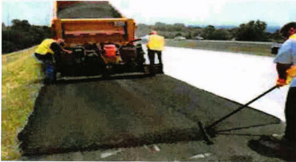
Typical asphalt installation
